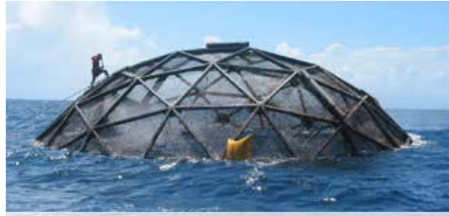
Aquapod: offshore pen for remote, offshore aquaculture / innovasea.com
